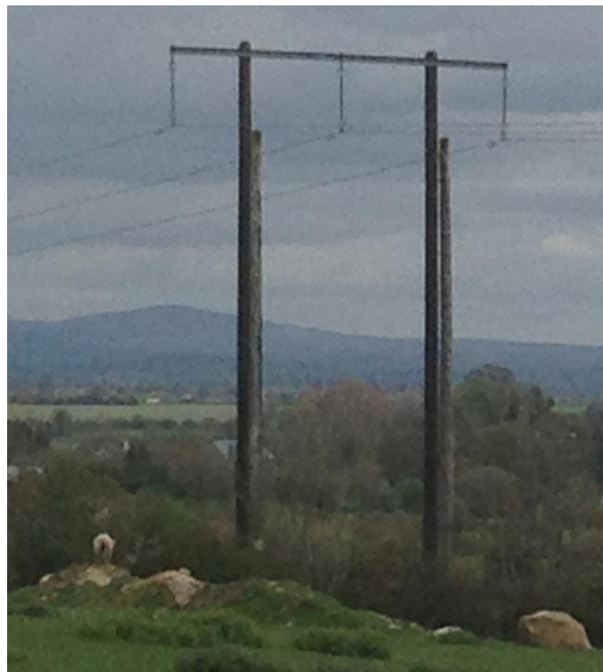
Figure 2-1: Example of existing 110 kV poleset being replaced with new and, in this instance, taller poleset (old poles still to be removed)
