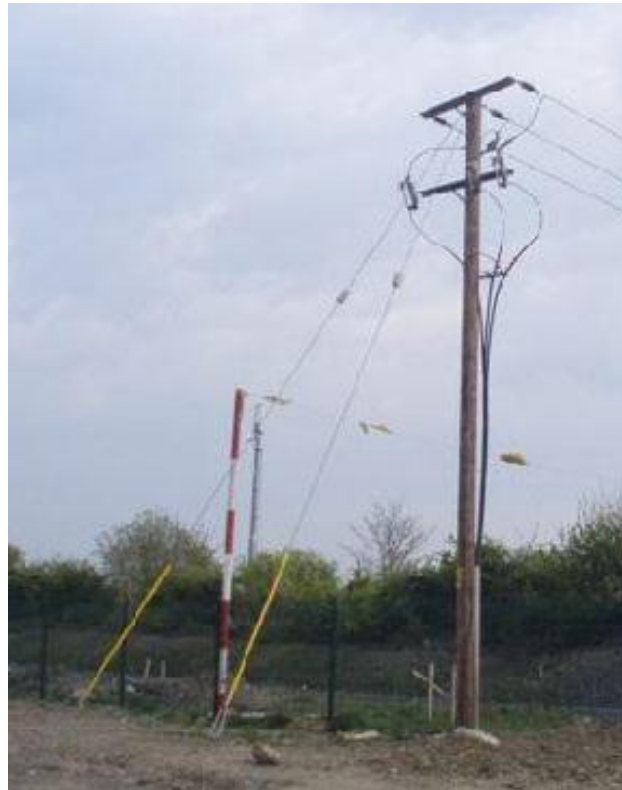
Figure 3-1: A typical MV line/cable interface pole
