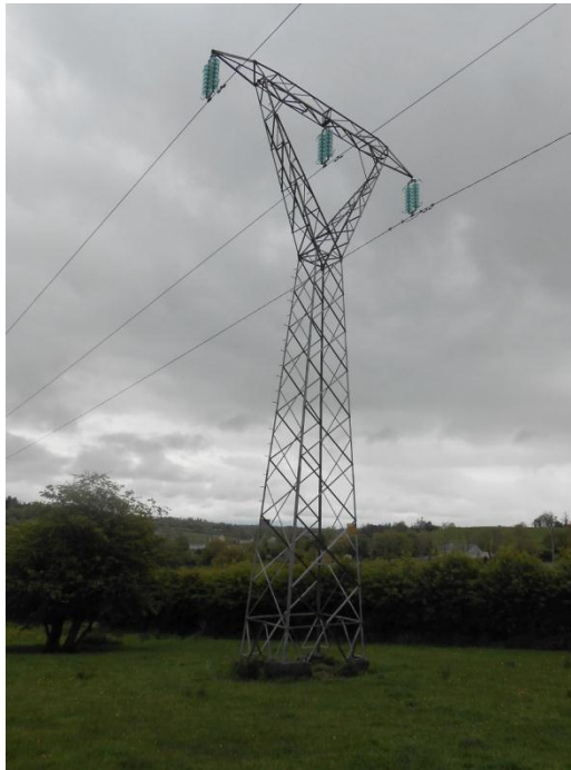
Figure 2-4: Example of a typical 110 kV Intermediate Lattice Steel Tower
